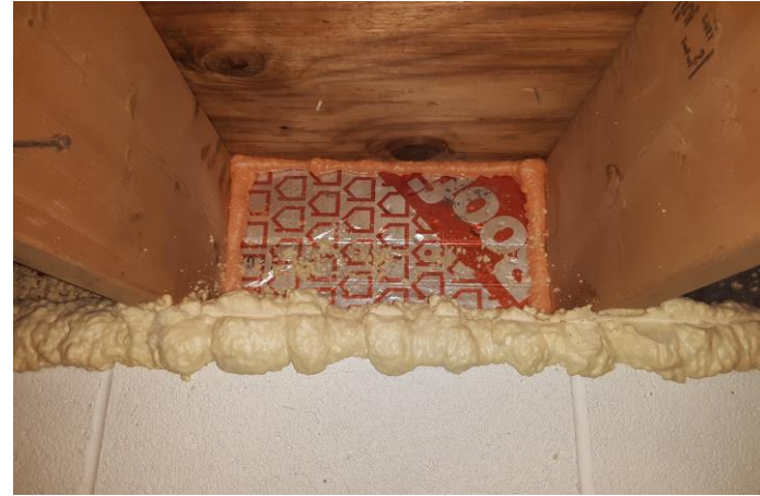
Rim joist air-sealing and insulation detail
