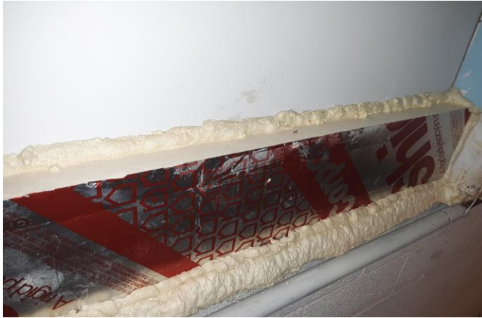
Rim joist air-sealing and insulation detail
